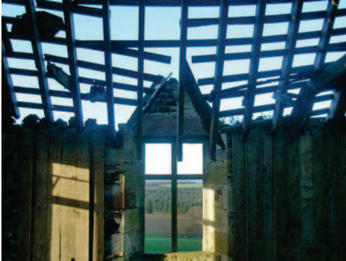
Above and below: Extensive damage to the roof has caused Fatlips to continue to deteriorate over the years. Above right: Fatlips at night. Photos contributed by Gemma Hon Turnbull Barnard.
